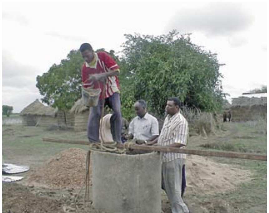
Brunnenbau in Ambe Banaan
